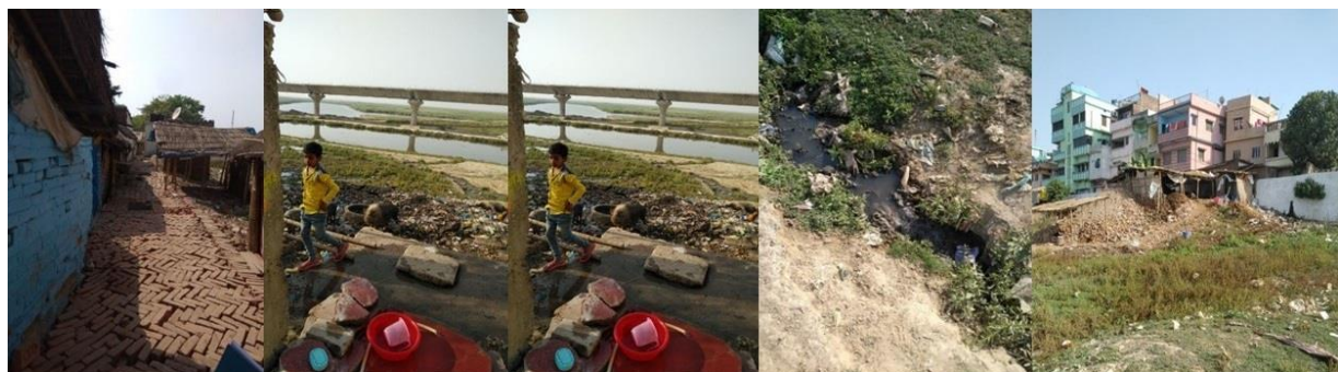
Figure 5: Encroached settlements, River edge, Waste water disposal and residential settlement
